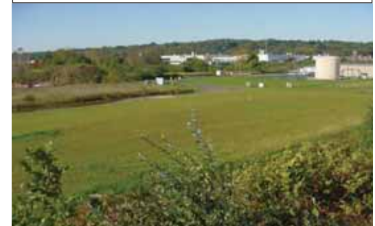
Photo 6. Completed final cover.
