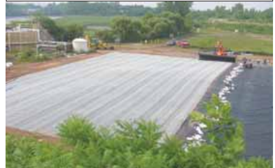
Photo 5. Geomembrane installation.
