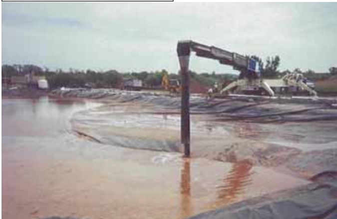
Photo 4. Placement of soil.
