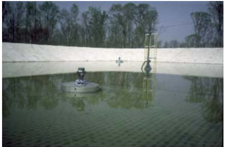
Photo 2. Fabri-form protected liner in an environmental pond.
